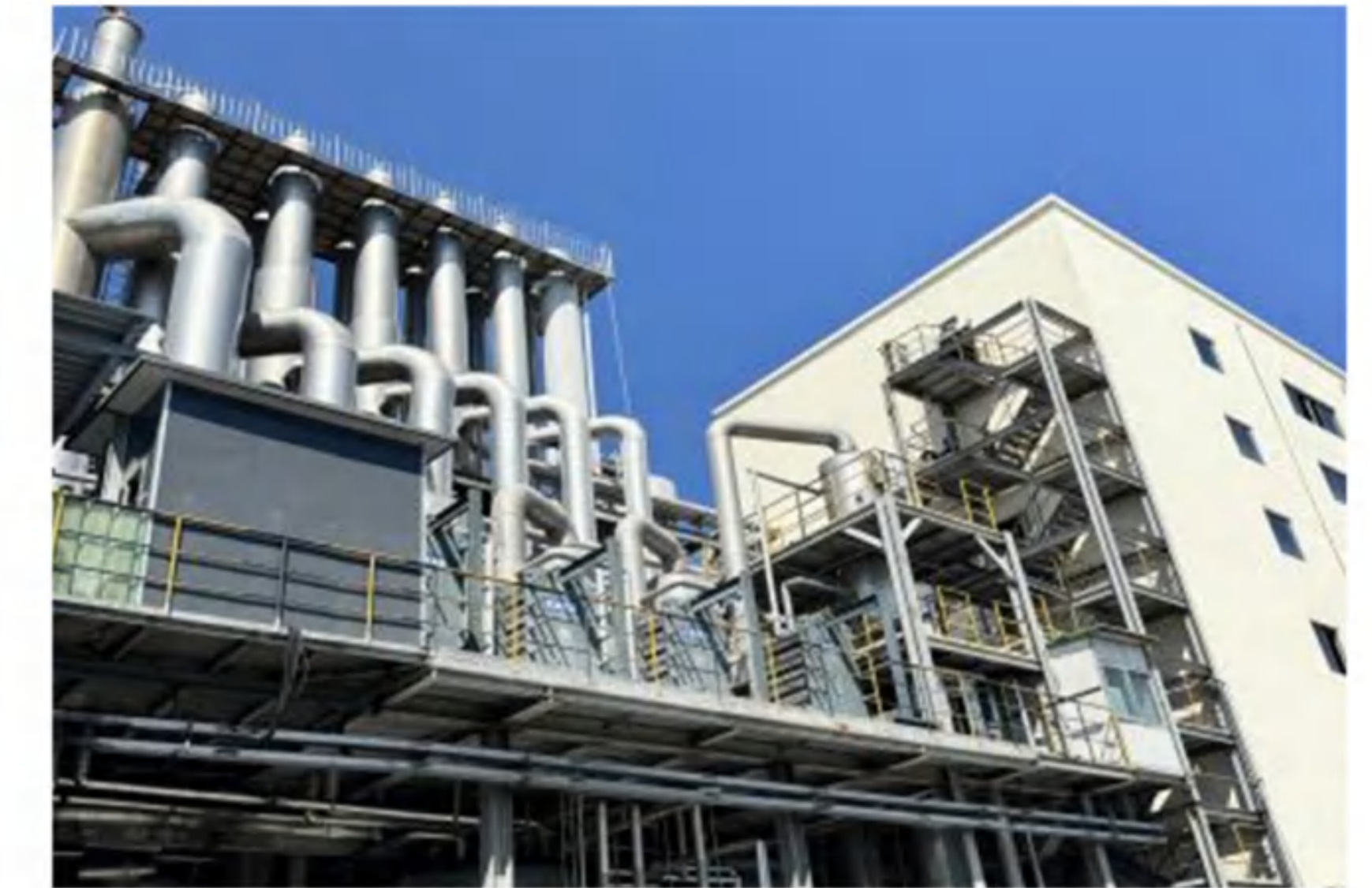
Evaporation: 5t/h Evaporation process: three-effect plate rising film + single-effect tube cross-flow process Materials: Monopotassium phosphate Final concentration: 60% Main material: TA1 TA2
