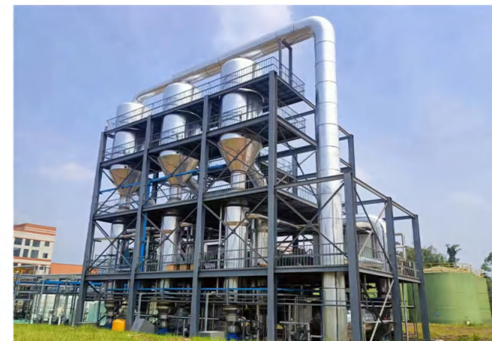
Evaporation capacity: 46.6t/h Evaporation process: triple effect tube+MVR forced circulation Material: Lithium sulfate Final concentration: crystallization Main material: SS316L
