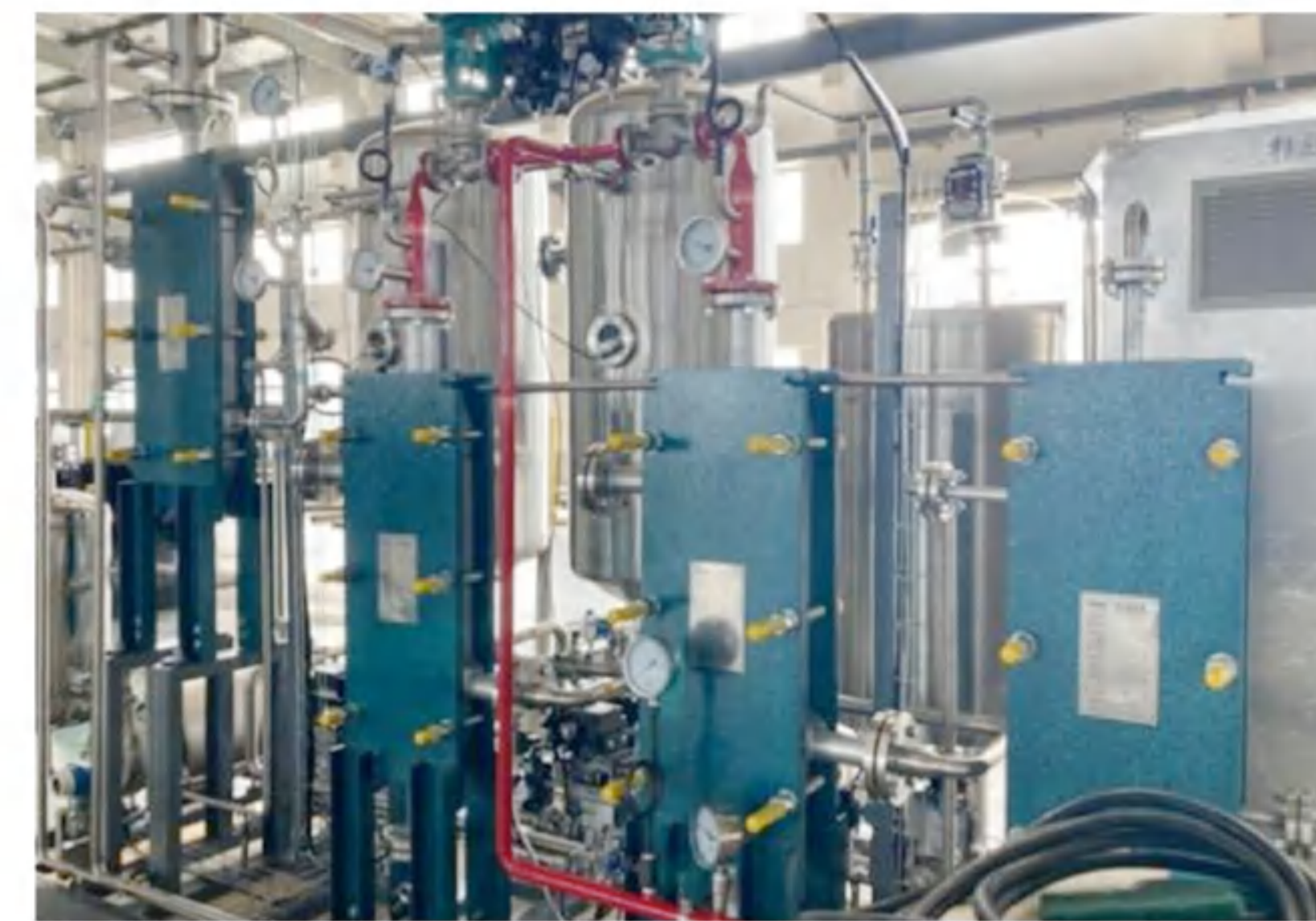
Evaporation capacity: 2.5t/h Evaporation process: Two effect Fluid: Oil Final concentration: 99.5% Main material: SS304
