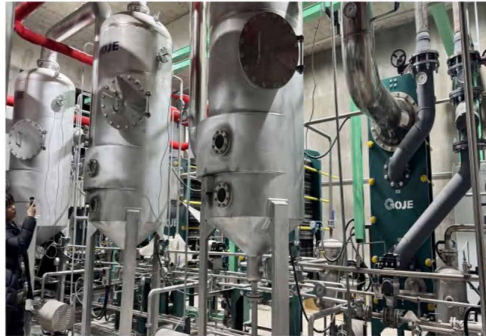
Evaporation: 4t/h Evaporation process: three-effect plate + TVR Ingredients: protein chondroitin Discharge concentration: 70% Main material: TA1
