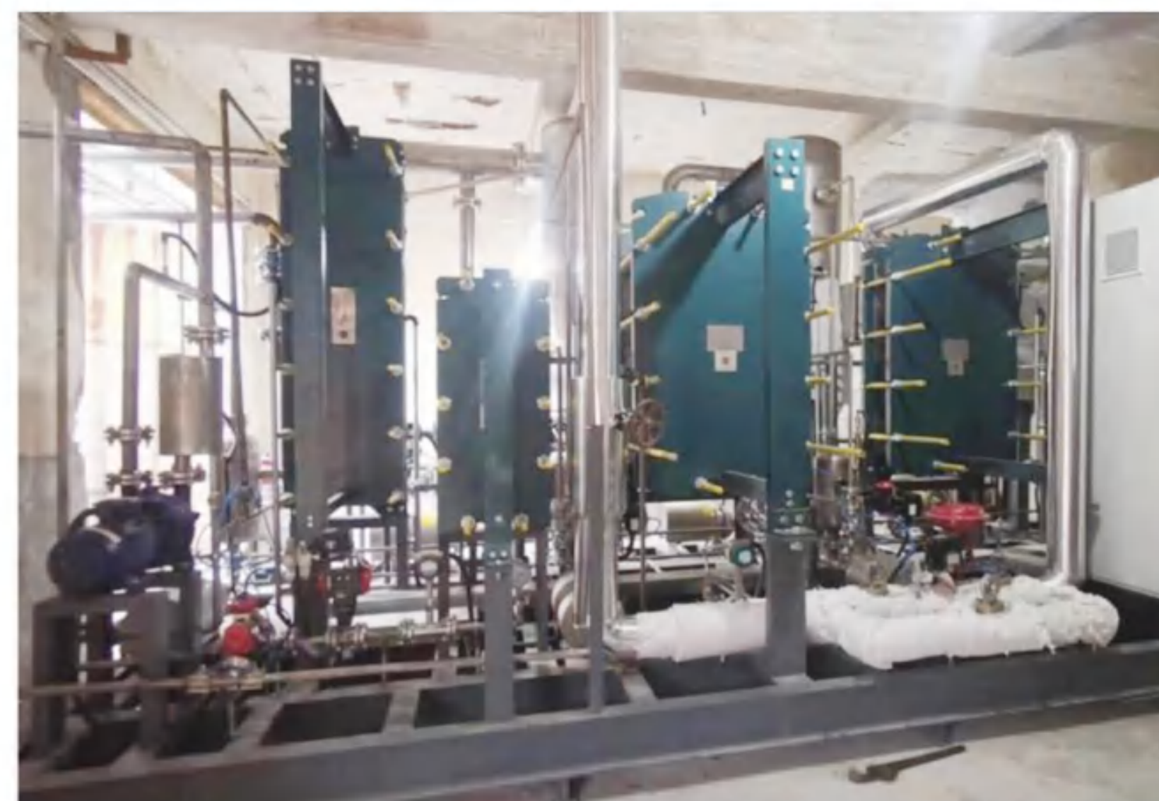
Evaporation capacity: 1.77t/h Evaporation process: Multi effect evaporation system Fluid: Glycerin Discharge concentration: 80% Main material: S30408
