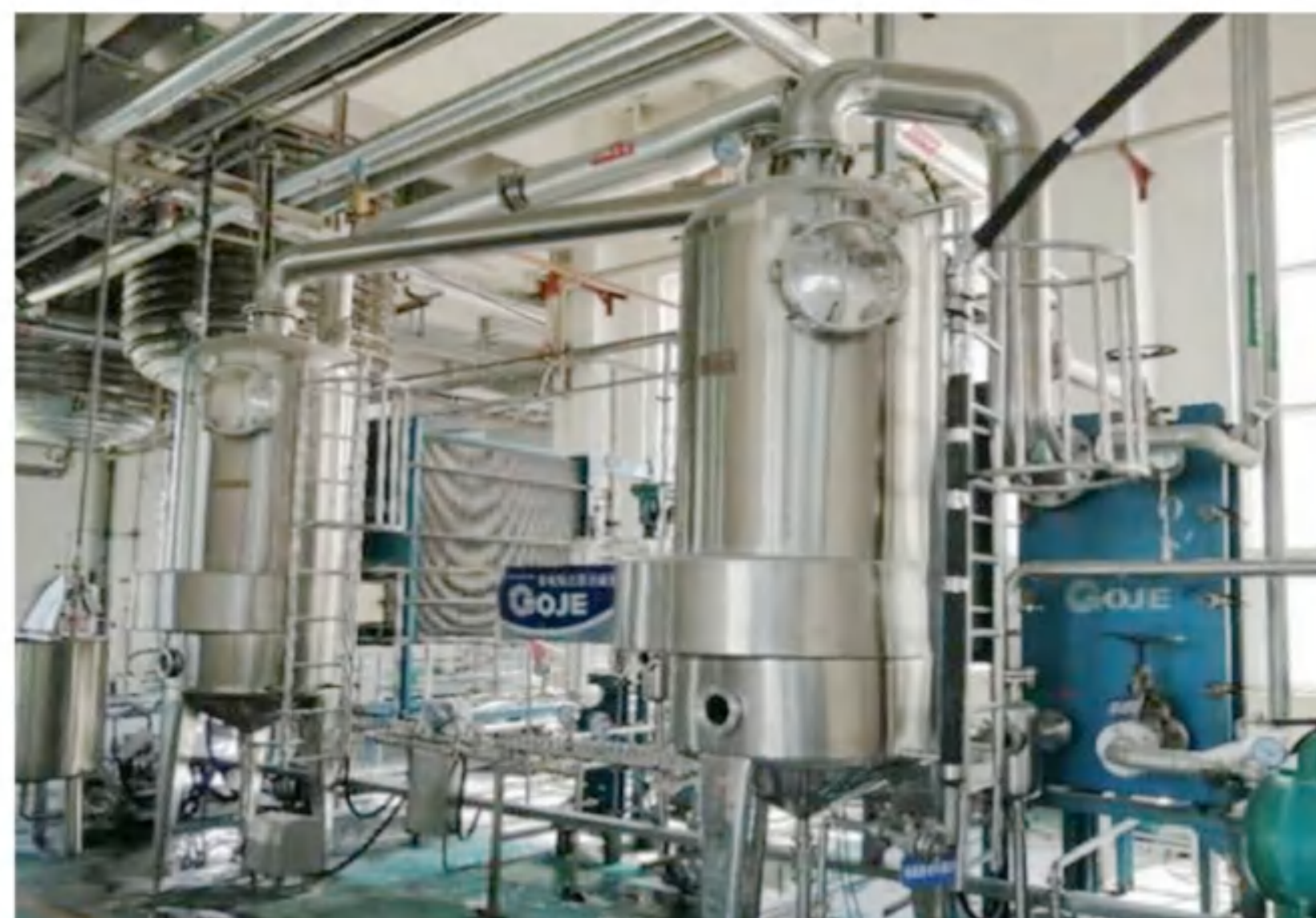
Evaporation capacity: 2t/h Evaporation process: Two effect TVR Fluid: Tartaric acid Final concentration: 50% Main material: SS316L
