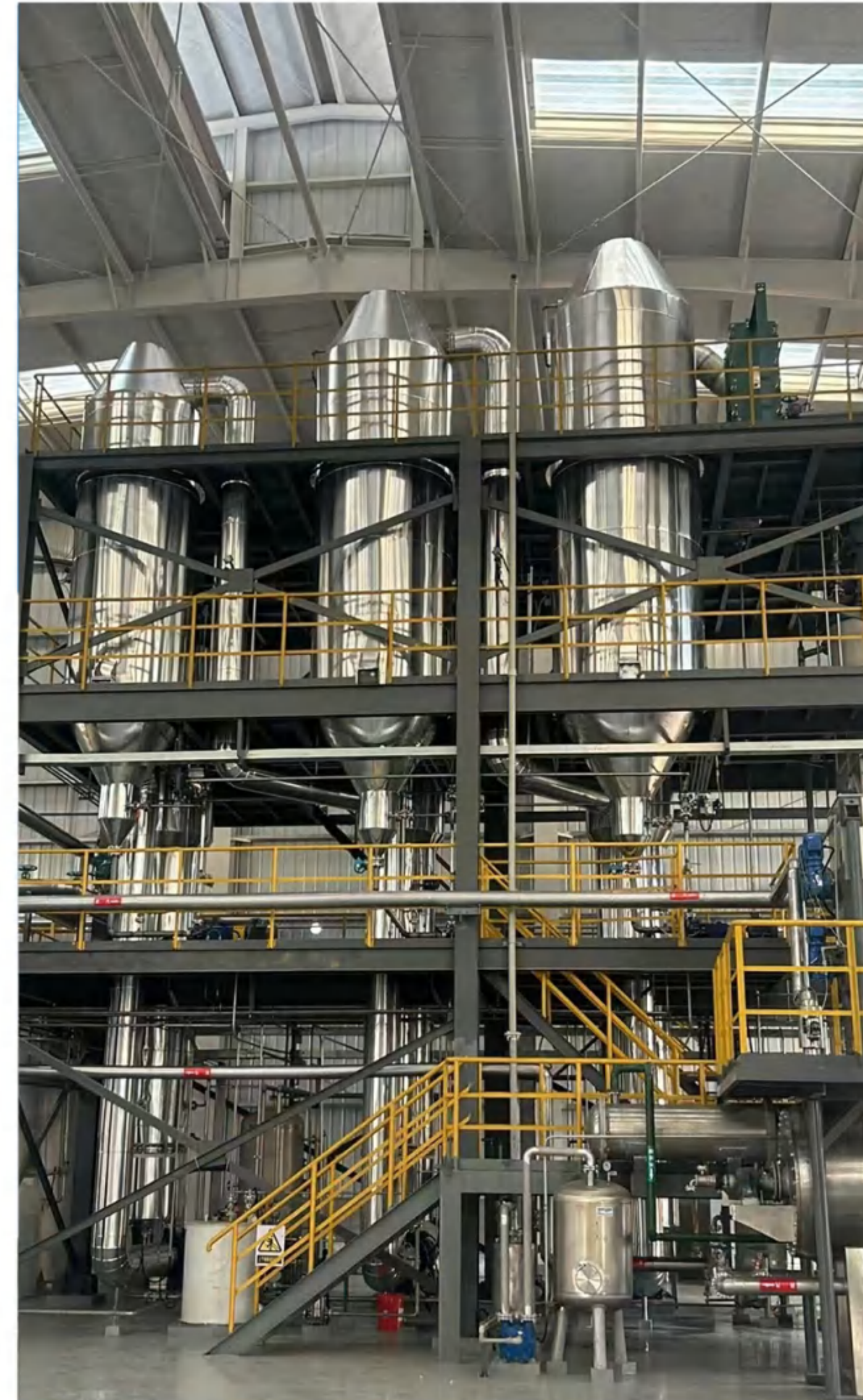
Evaporation: 4.5t/h Evaporation process: MVR tube falling film + forced circulation Ingredients: potassium chloride Final concentration: Crystallization Main material: TA1 TA2
