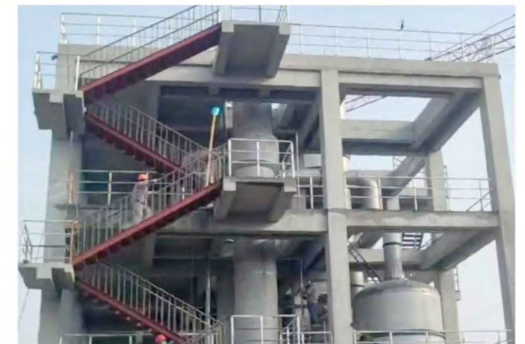
Evaporation capacity: 41t/h Evaporation process: Two effect falling film+MVR forced circulation Material: Sodium sulfate Final concentration: 28% Main material: SS316L
